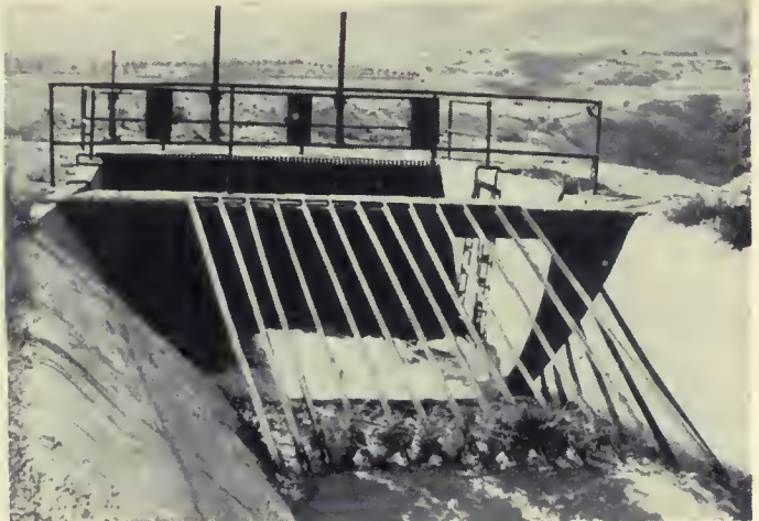
STEEL BARS DO NOT A PRISON MAKE —they are a means of escape from canals. Above, reinforcement bar mats and an escape ramp on the side slopes of the North Branch Canal, Kittitas Division, Yakima project, Washington. At right, handrails and escape ladders at the Jordan Narrows siphon of the Provo River project, Utah. Photo above by S. T. Larsen, Denver, Colo.; at right by R. W. Reitz, Region 4.
